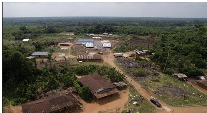
Figure 2: Obayantor community aerial view
