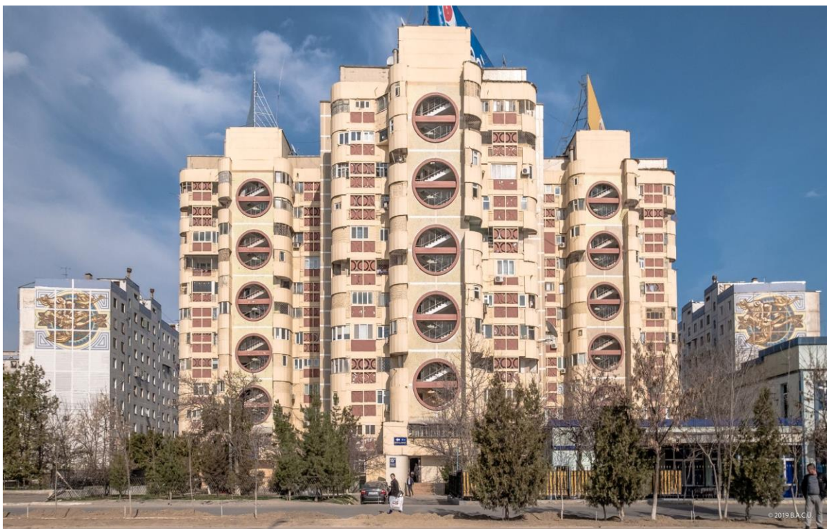
Picture 3: Residential apartments, Tashkent, Uzbekistan, Built in the 80s. Architect Victor Breusenko.
