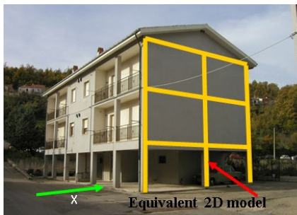
Fig. 3. Bonefro reinforced concrete 3-storey building
