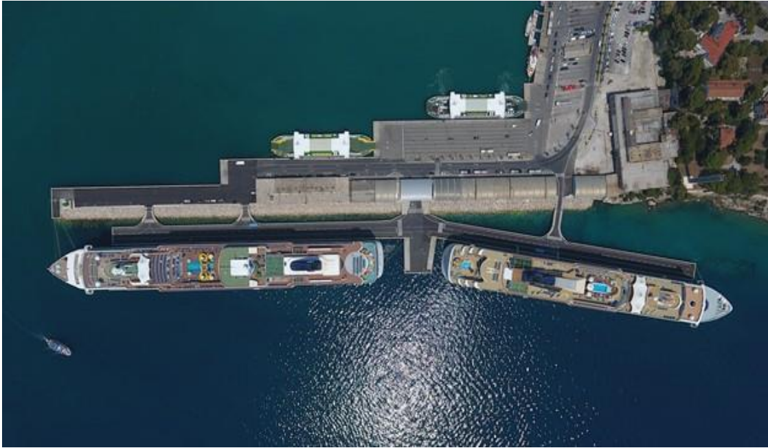
Figure 3: Newly constructed coastal area with operational moorings [4]
