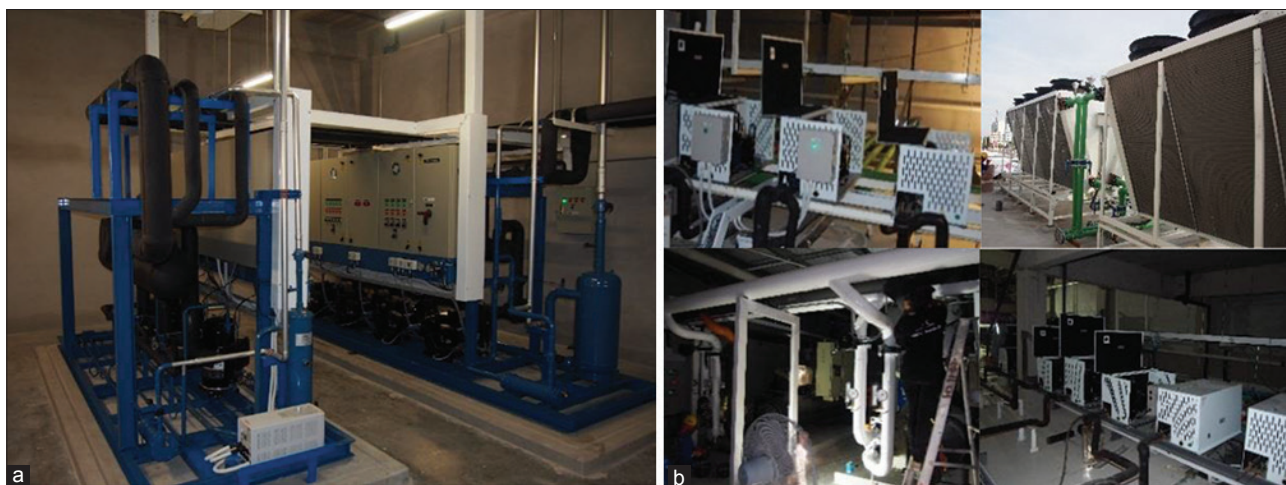
Figure 8: Those are elements of 2 types of refrigeration system: (a) Conventional multi set rack (b) Water loop system
