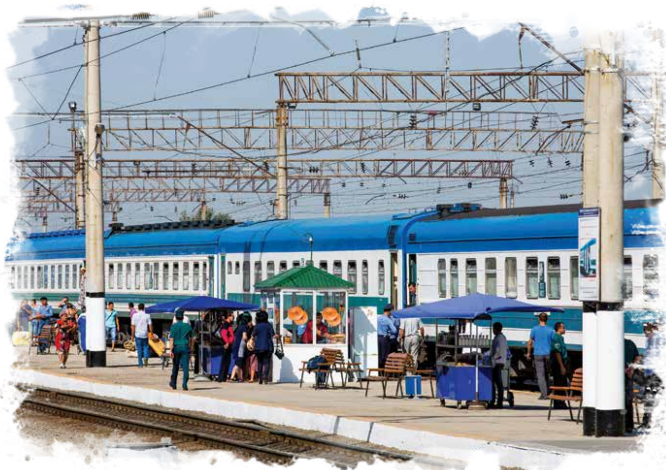
Samarkand Railway Station, Uzbekistan. The north–south corridor linking Europe through Central Asia to the Middle East and South Asia passes through Samarkand City in Uzbekistan. ADB assisted in the electrification of 140 kilometers of this railway line, which annually carries about 10 million tons of freight (photo by Relisa Granovskaya for ADB).
