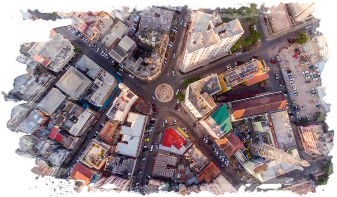
Dar es Salaam. Tanzania's largest city is an economic hub in East Africa and requires significant infrastructure investments to handle the continuous influx of new migrants to its expanding urban and peri-urban areas (photo by Moiz Husein/iStock.com).
