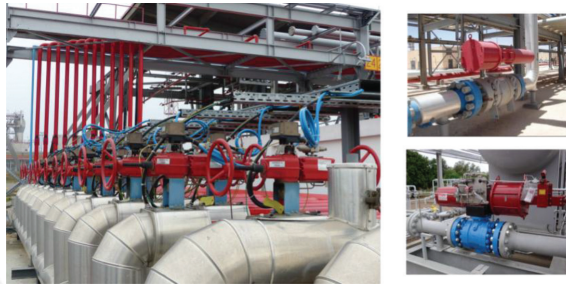
Figure 7. Example of emergency shutdown valve.
