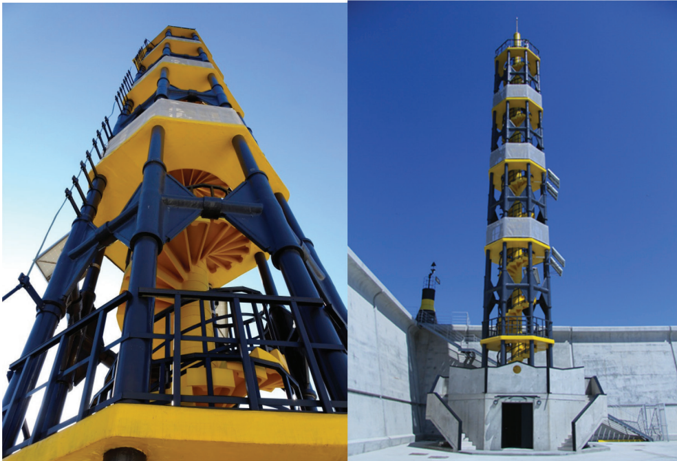
Figure 8. The FRP lighthouse (Valencia, Spain): Left: lighthouse detail, Right: general view of the lighthouse in Port of Valencia.
