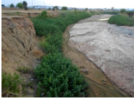
Fig. 11. Carnea transplanted away from the stream bank to curtail expansion of fluvial erosion
