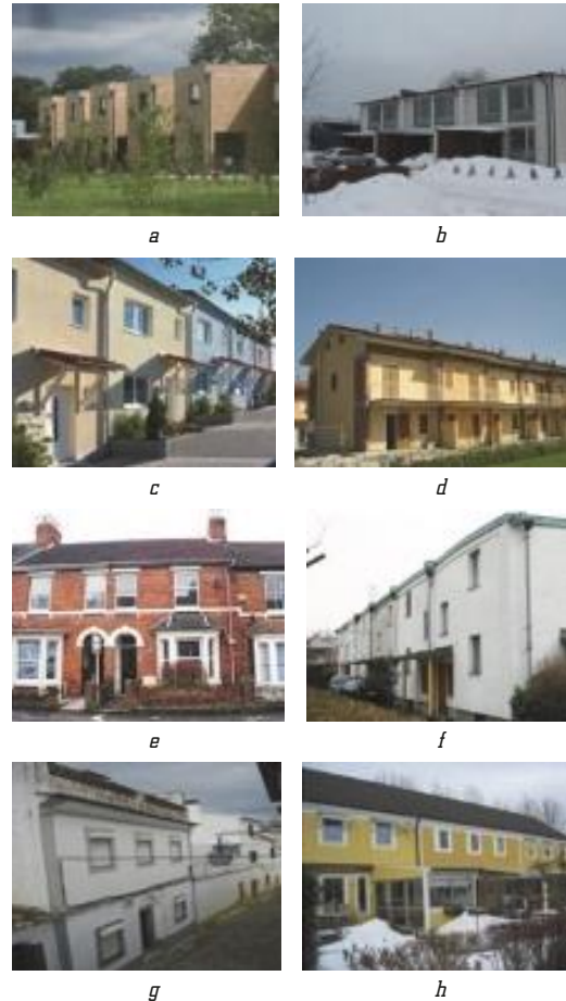
Fig. 2. Examples of buildings: a, c-h – a townhouse in a classic form; b – duplex townhouse
