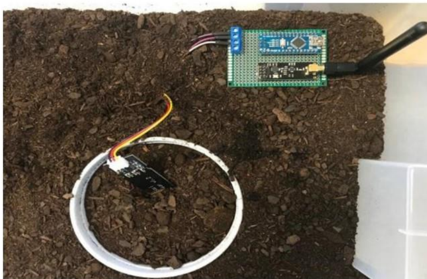
Figure 11 Substation in real set.
