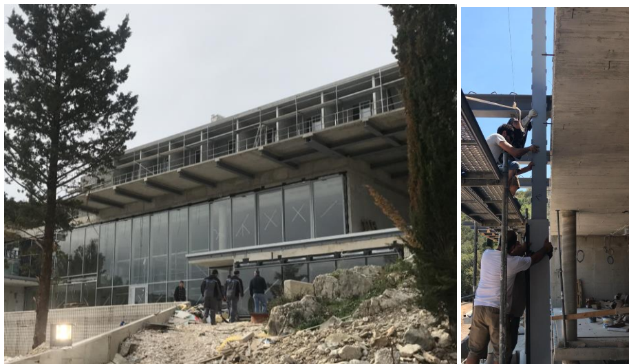
Figure 10 Glass facade of Hotel Osmine in Slano
