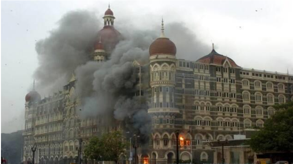
Figure 4: Taj Mahal Hotel, Mumbai, attacked by terrorists in 2008 (Source: The Indian Express (2023))
