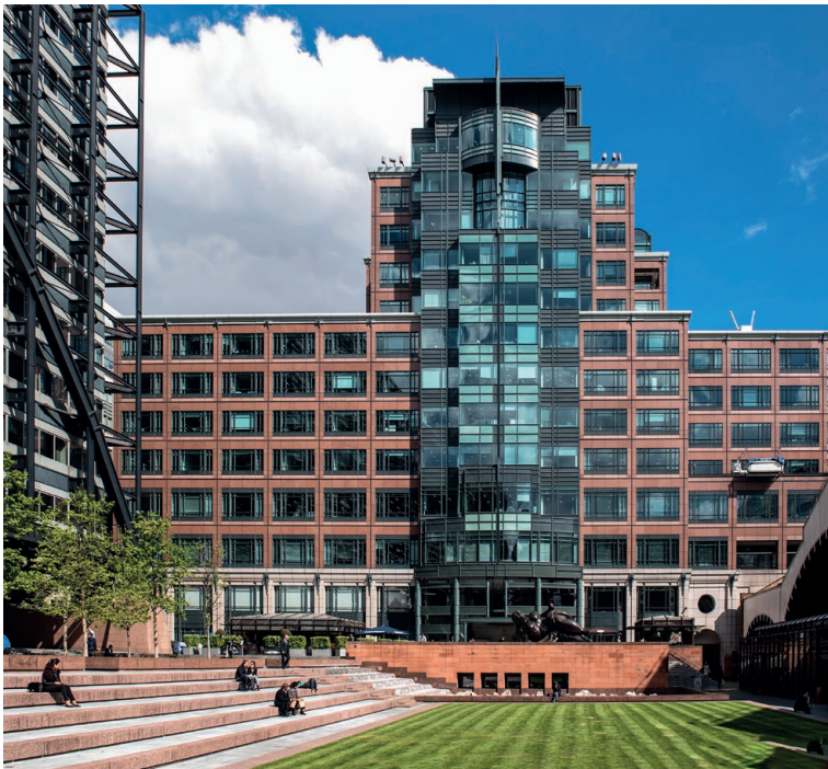
The EBRD's new London Headquarters opens at One Exchange Square in March 1993
